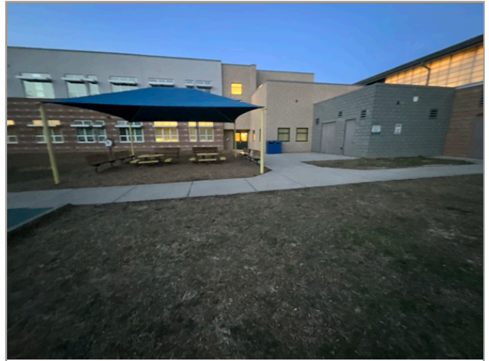
ACCESSIBLE ROUTE TO PLAYGROUND
