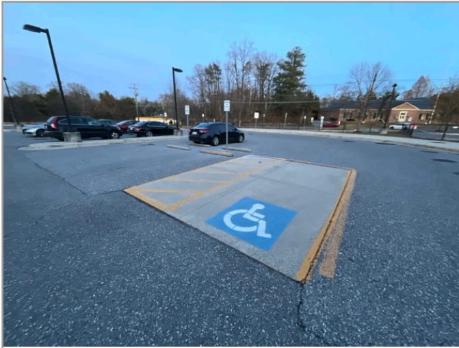
OVERVIEW OF ACCESSIBLE PARKING AREA
